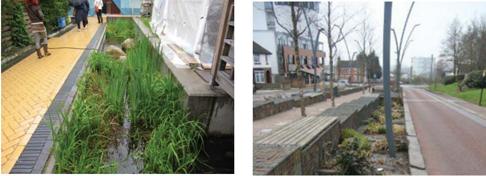
Figure 13. Bioretention areas in the cities
