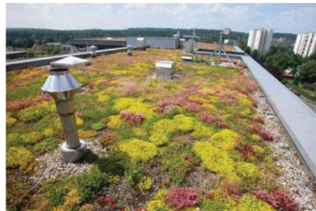
Figure 5. Extensive green roof
