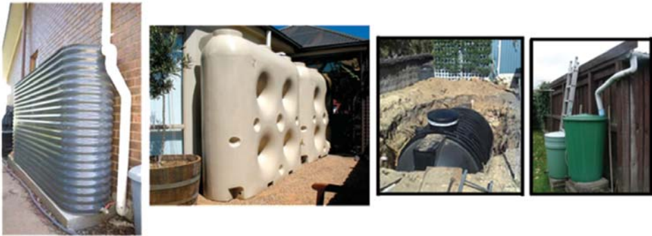
Figure 7. Tanks for rain harvesting
